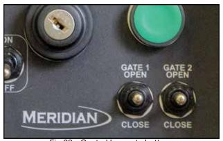
Fig 39 - Control box gate buttons
